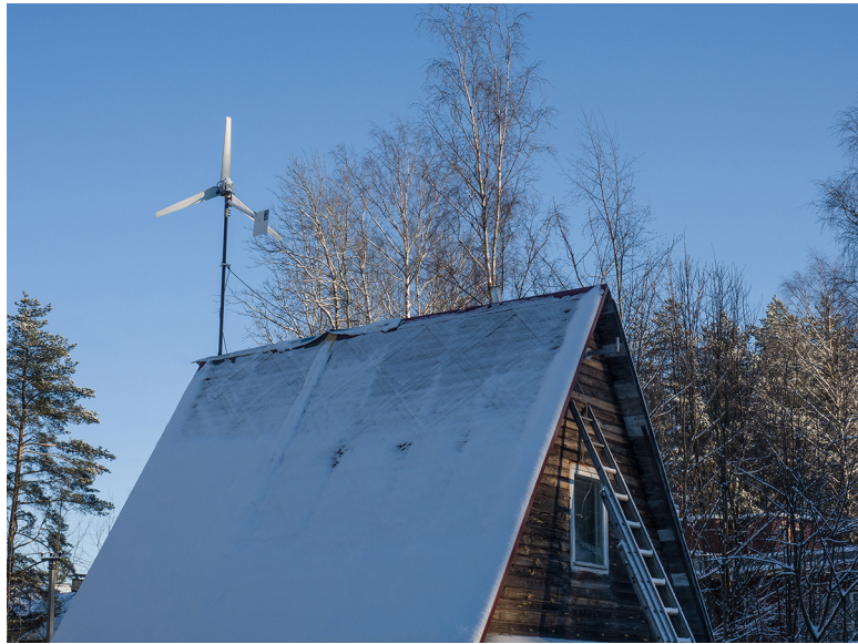
Figure 17. Cabin powered by a stand-alone wind power system.
